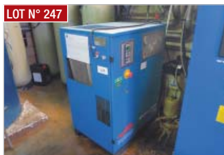
▶ Compresseur WORTHINGTON CREYSSENSAC , type RLR 1500BM7 ▶ WORTHINGTON CREYSSENSAC Compressor , type RLR 1500BM7
