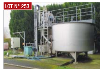
▶ Station de prétraitement des eaux usagées ▶ Waste water pre-treatment plant
